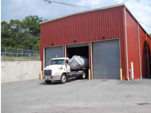
LIQUID SLUDGE OFF LOAD BUILDING
